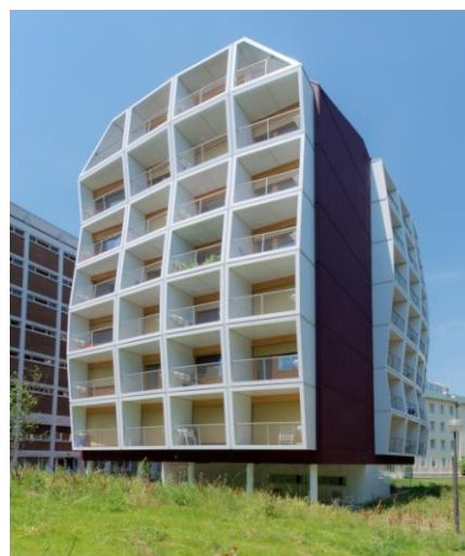
Paris, France Wooden 7 multi-storey building Carbon storage: ca. 1,200 tonnes Construction time 4 months
